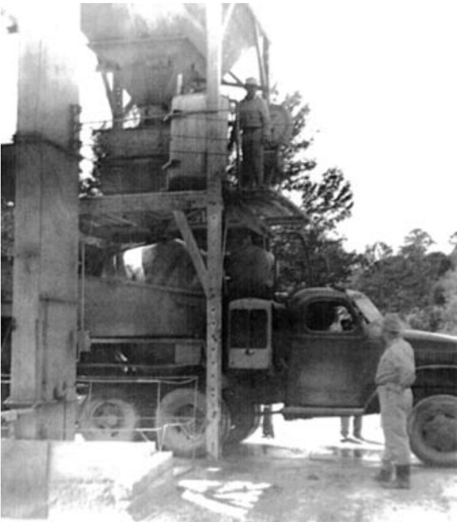
Fig. 2: In the 1950s, a surplus WWII army truck carried a 4-yd<sup>3</sup> (3-m<sup>3</sup>) mixer
